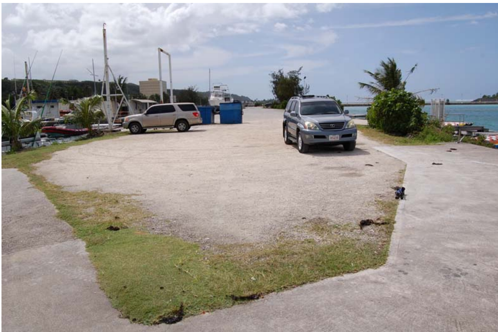
Westerly view along subject marina dry dock area. The outer basin area is to the right.
