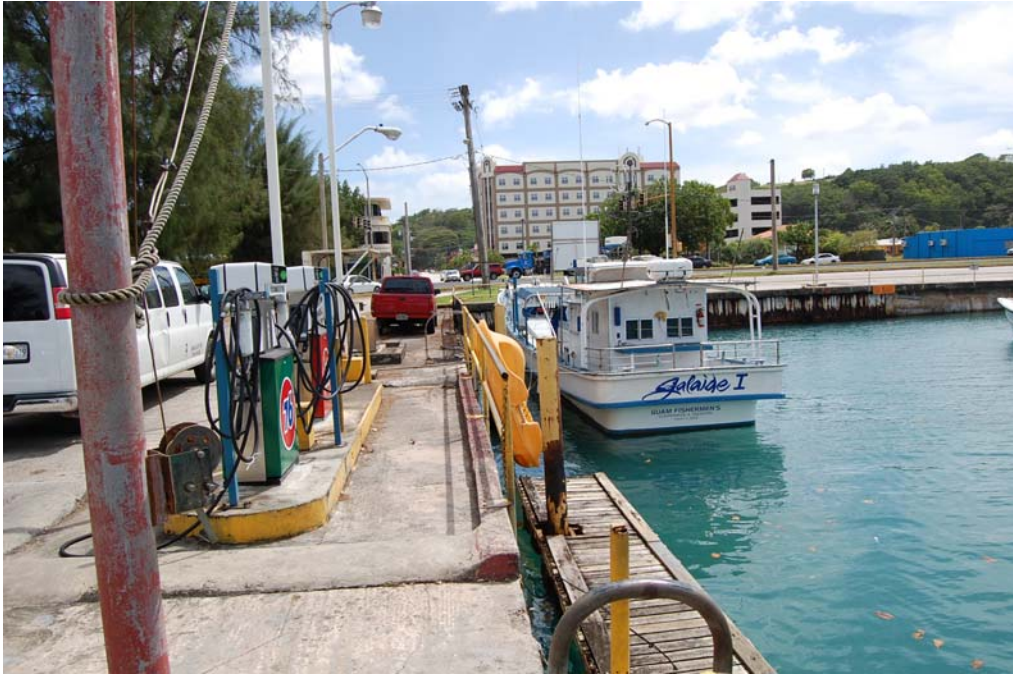
View of the nearby Guam Fishermen's Cooperative Association fuel pier.
