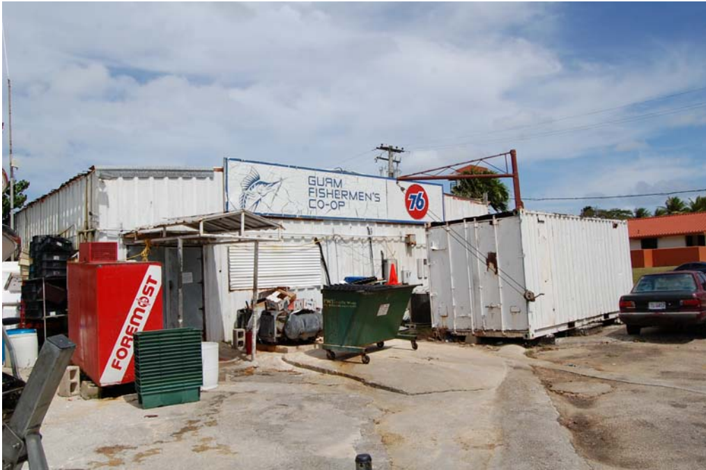
Northeasterly view at Guam Fisherman's Cooperative Association improvements. Note the metal butler style building construction.
