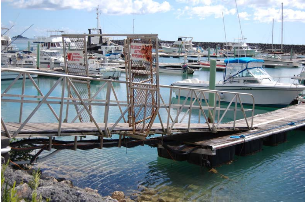
View of gangway area with security gate.
