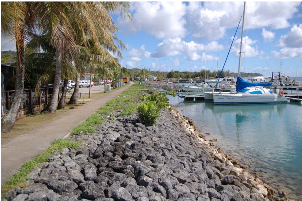
Southerly view along interior revetment rock wall and marina water frontage.
