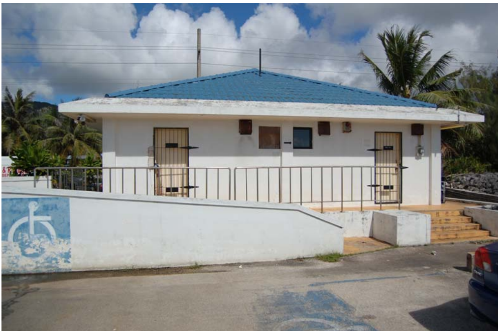
View of closed restrooms one-story concrete building.
