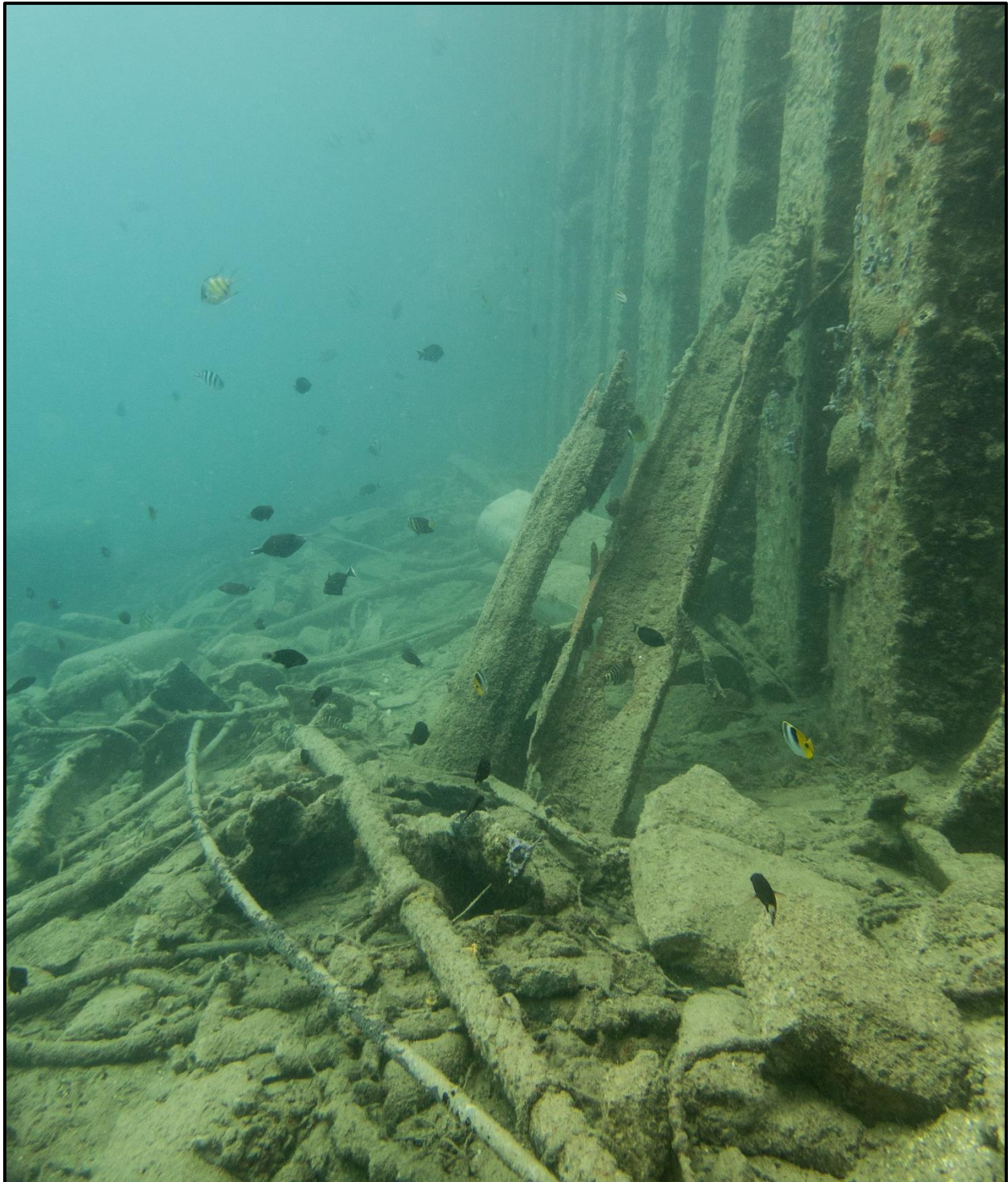
Figure 29. A portion of the debris field occurring at the base of the south wharf face at a depth of approximately 9 m. The debris are strewn across a seafloor dominated by uncolonized, unconsolidated sediment, but some coral colonies were observed growing on the debris.
