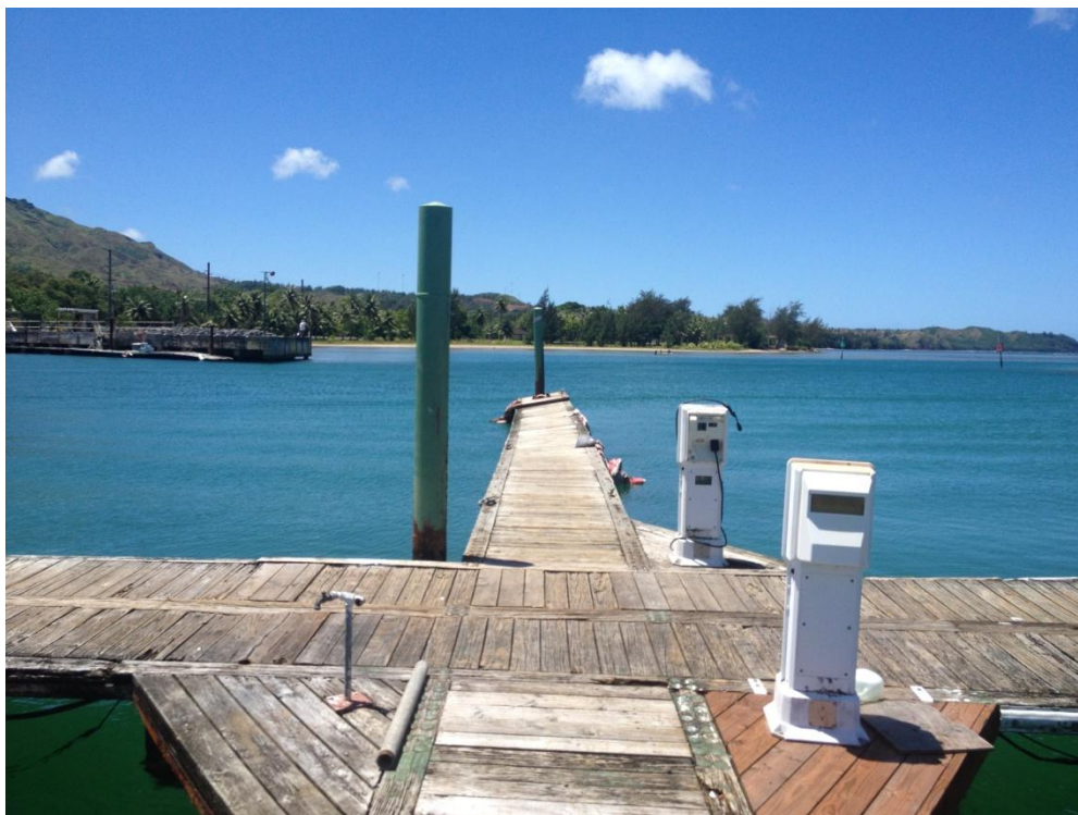
Photo Description: Looking south along finger off of main dock A.
