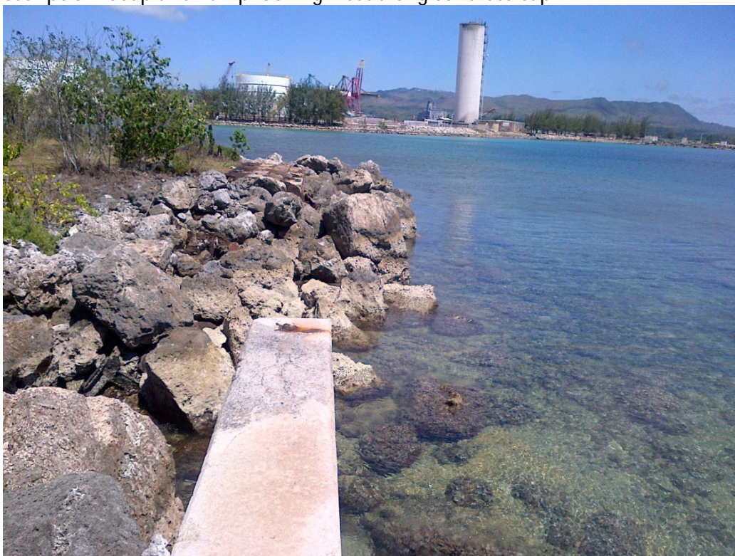
Photo Description: Seaplane Ramp looking east.
