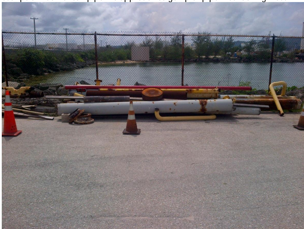
Photo Description: Pile of old piping near the gate from replacement work. Tenant considers this a PAG asset so they can't dispose of it.
