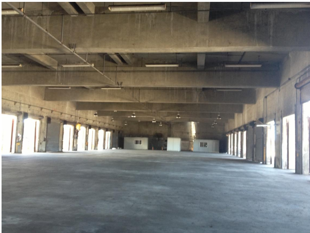
Photo Description: Interior of CFS building looking west.
