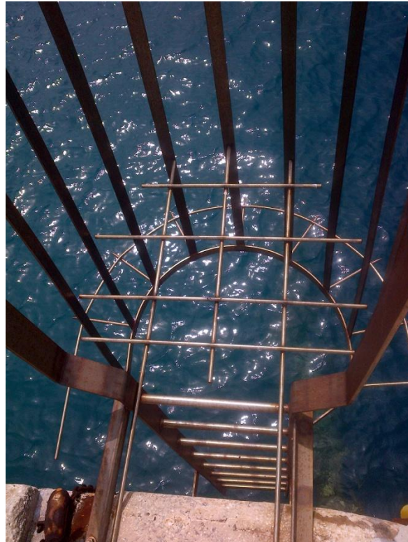
Photo Description: Fire escape from the eastern breasting dolphin.
