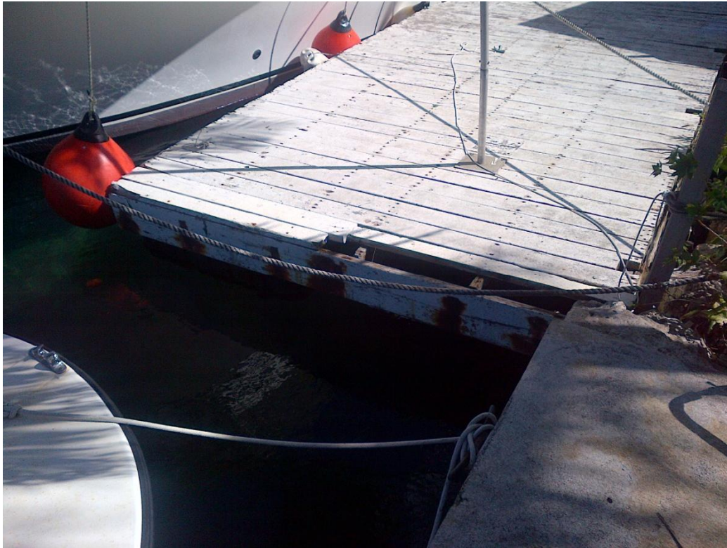
Photo Description: Dock at southwest end looking northeast.
