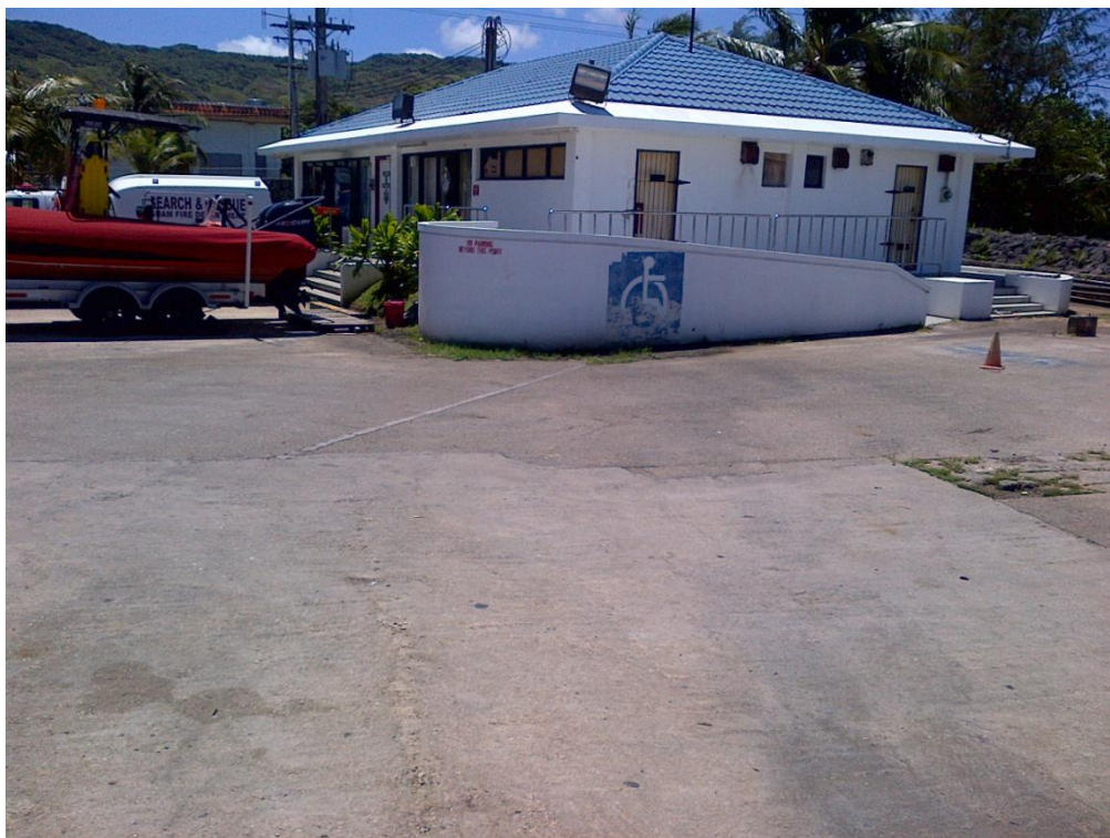
Photo Description: Agat Marina Administration Building looking southeast.
