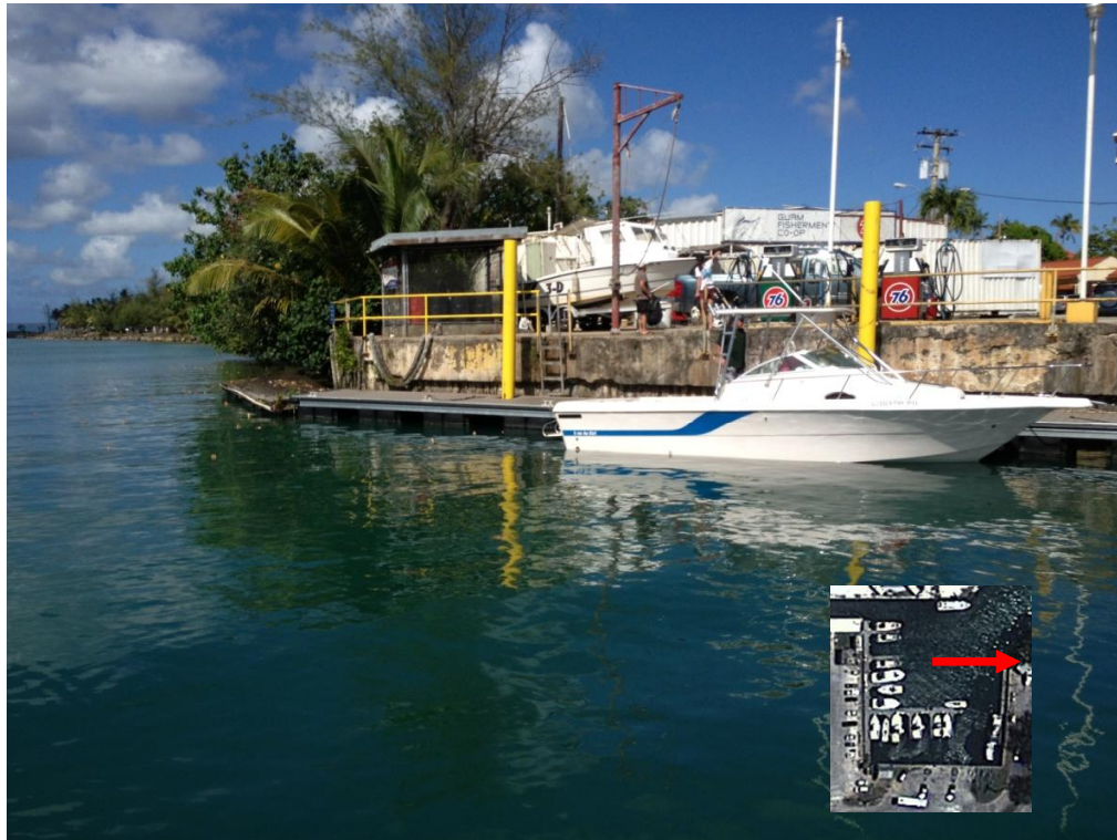
Photo Description: Fueling dock/ float on the eastern wall of the east basin of the marina looking east. Fuel pumps are not operated by PAG.
