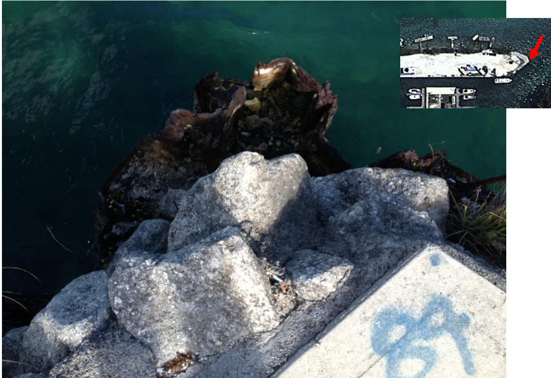
Photo Description: Sheetpile wall along entrance to the marina.
