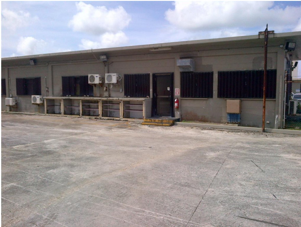
Photo Description: North side of the Tank Farm A administration building looking south.
