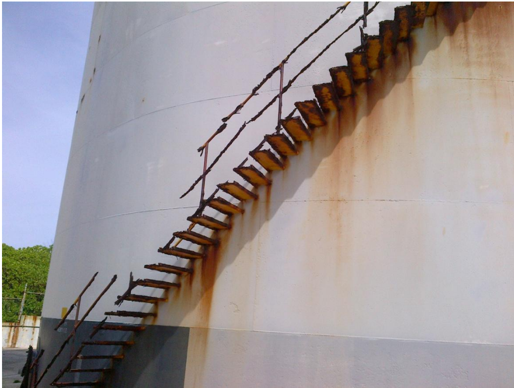
Photo Description: Tank 3 stairway looking northwest.
