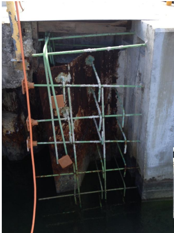
Photo Description: End of Phase 1 sheetpile replacement. Phase 2 is currently underway.
