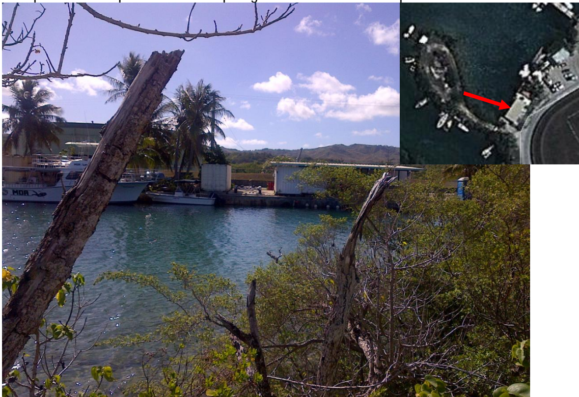
Photo Description: Photo of above concrete structure at a distance looking east.
