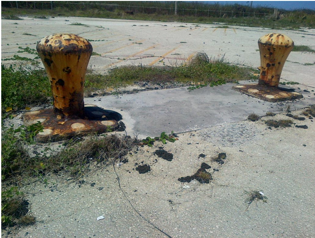
Photo Description: Landside bollards north of the Hotel Wharf structure.
