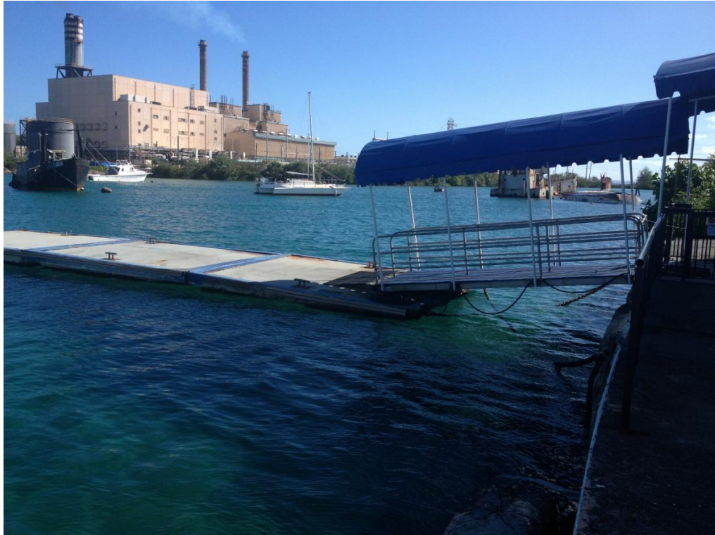
Photo Description: Dock at Aqua World looking northeast towards GPA's Cabras island power plant.
