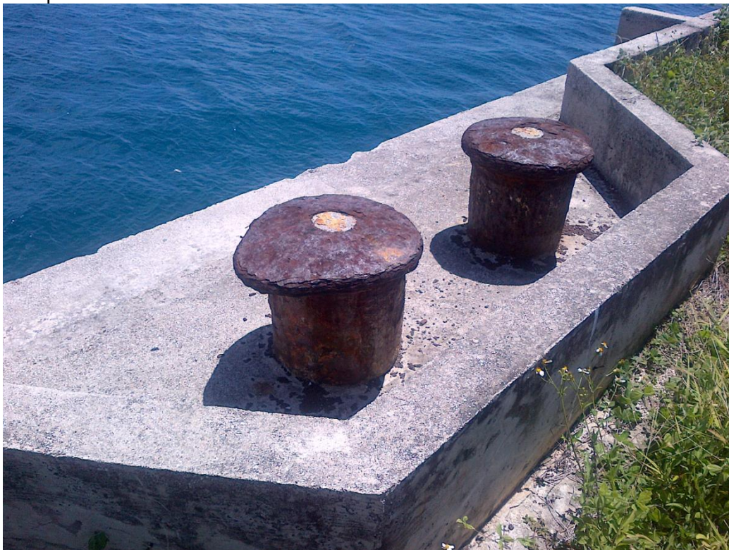
Photo Description: Cleat on the Hotel Wharf bulkhead structure.
