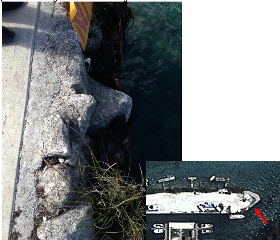
Photo Description: Sheetpile wall along entrance to the marina.
