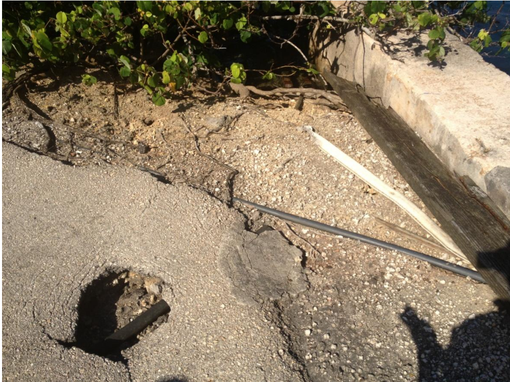
Photo Description: Sink hole forming behind bulkhead near Aqua World on the north edge of parking area.
