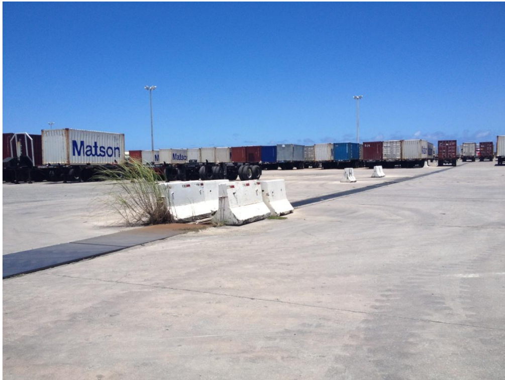
Photo Description: Trench drains on the eastern portion of the yard.
