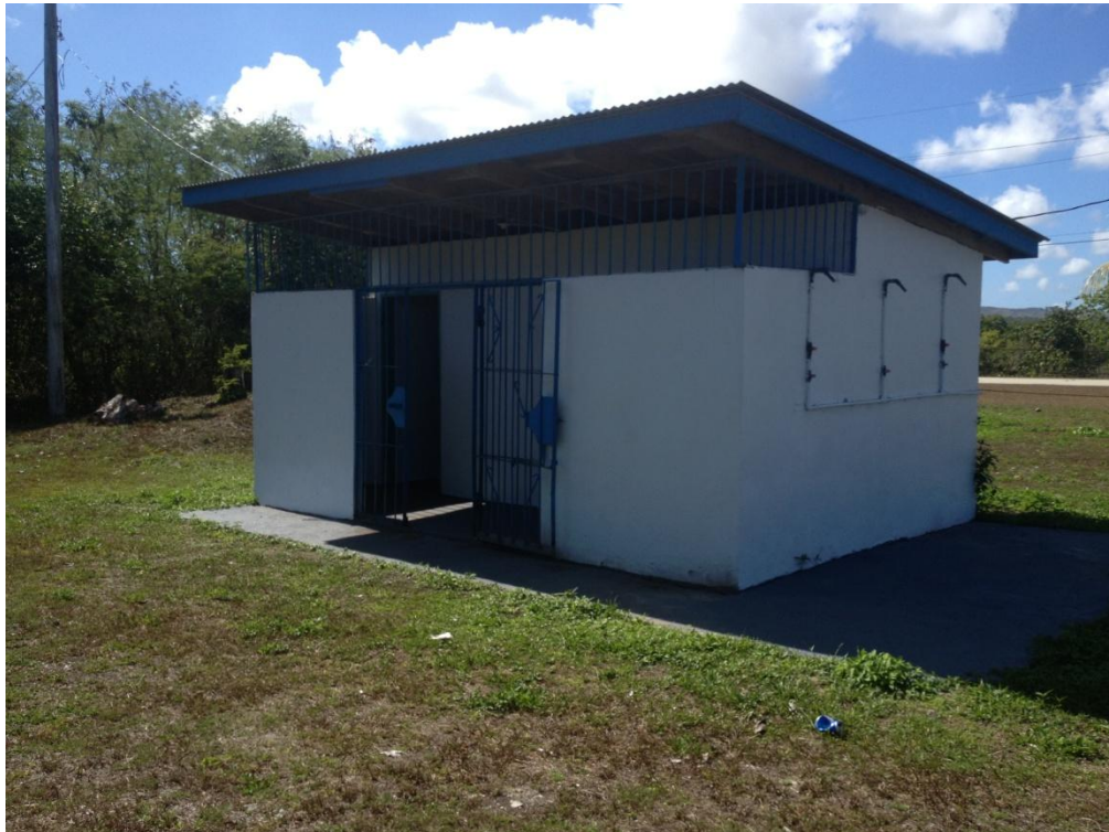
Photo Description: Restroom facility on the upper area looking southeast.
