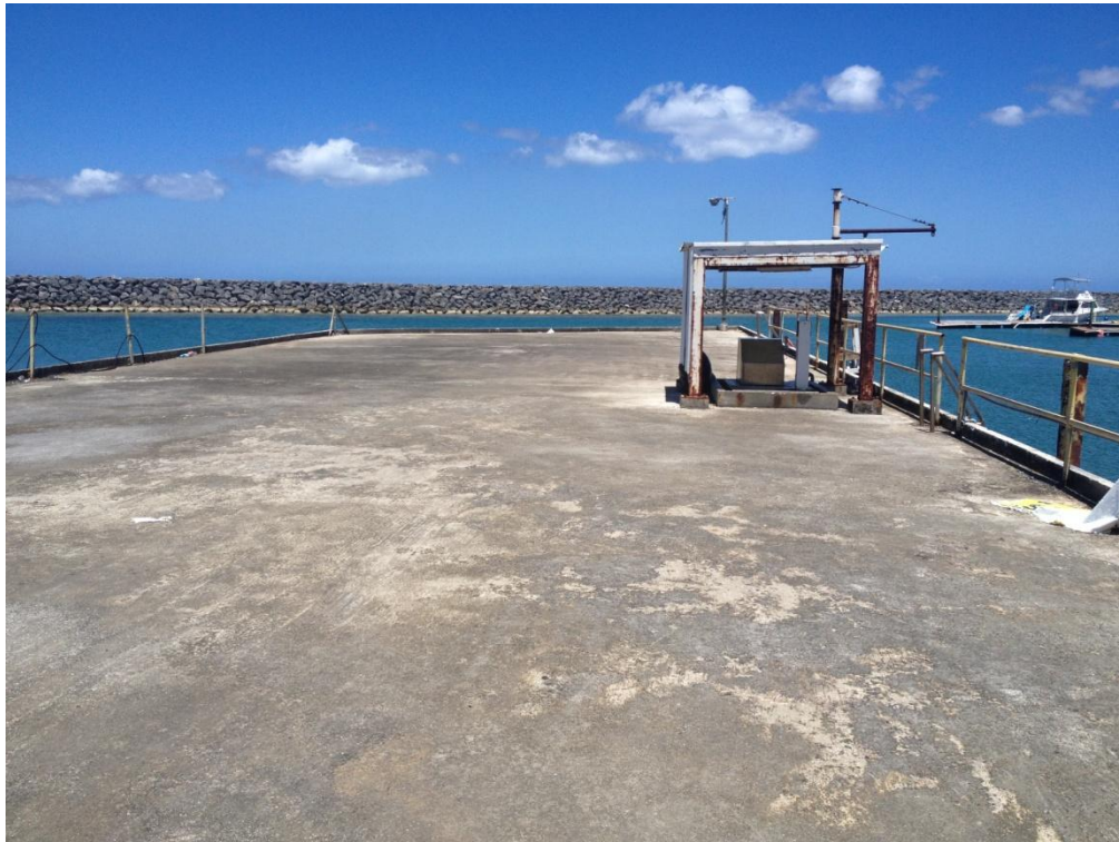
Photo Description: On top of elevated pier looking west.
