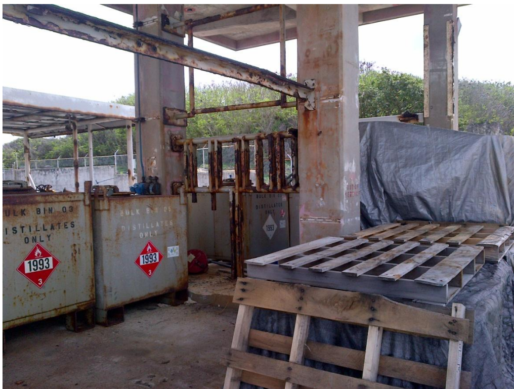
Photo Description: Closer photo of the loading rack looking northeast.
