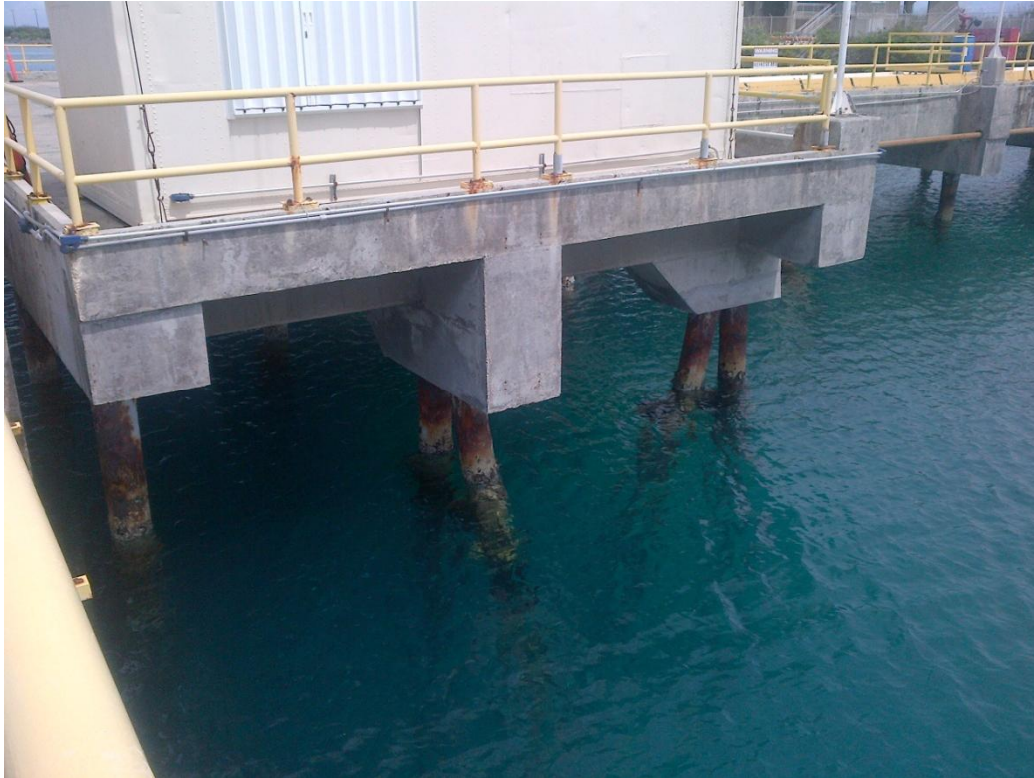
Photo Description: Main Pier Structure looking northwest from the eastern catwalk.
