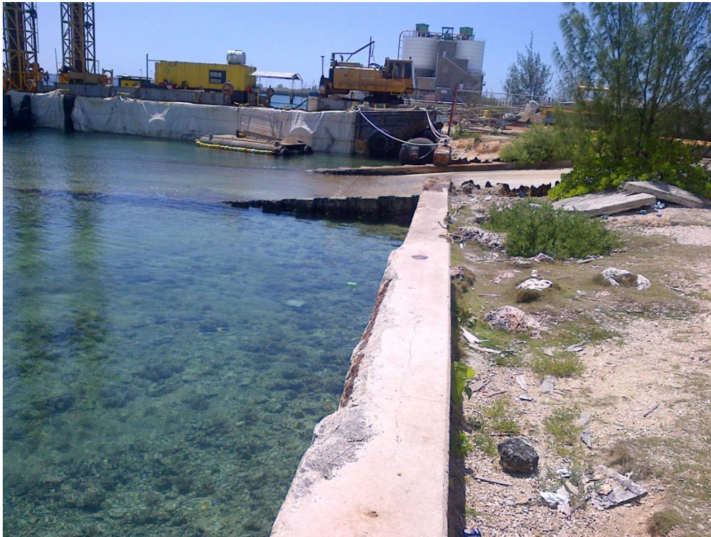
Photo Description: Seaplane Ramp looking west along concrete cap.
