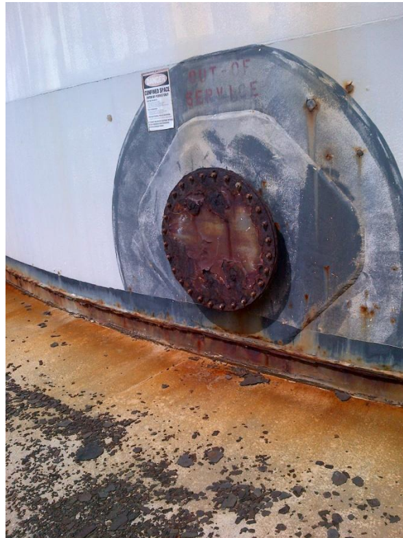
Photo Description: Tank 1 access cover on the northeast side.
