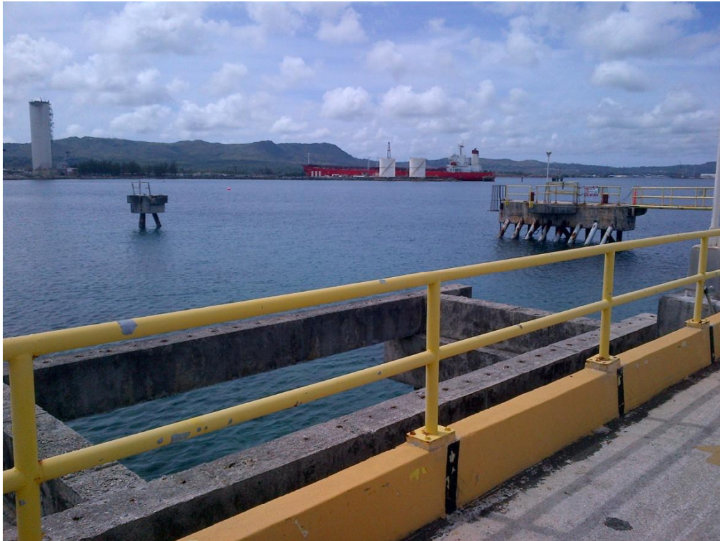
Photo Description: Breasting and mooring dolphins to the east of the Golf Pier main structure.
