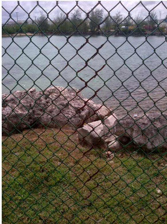
Photo Description: Fencing around Golf Pier (typical).
