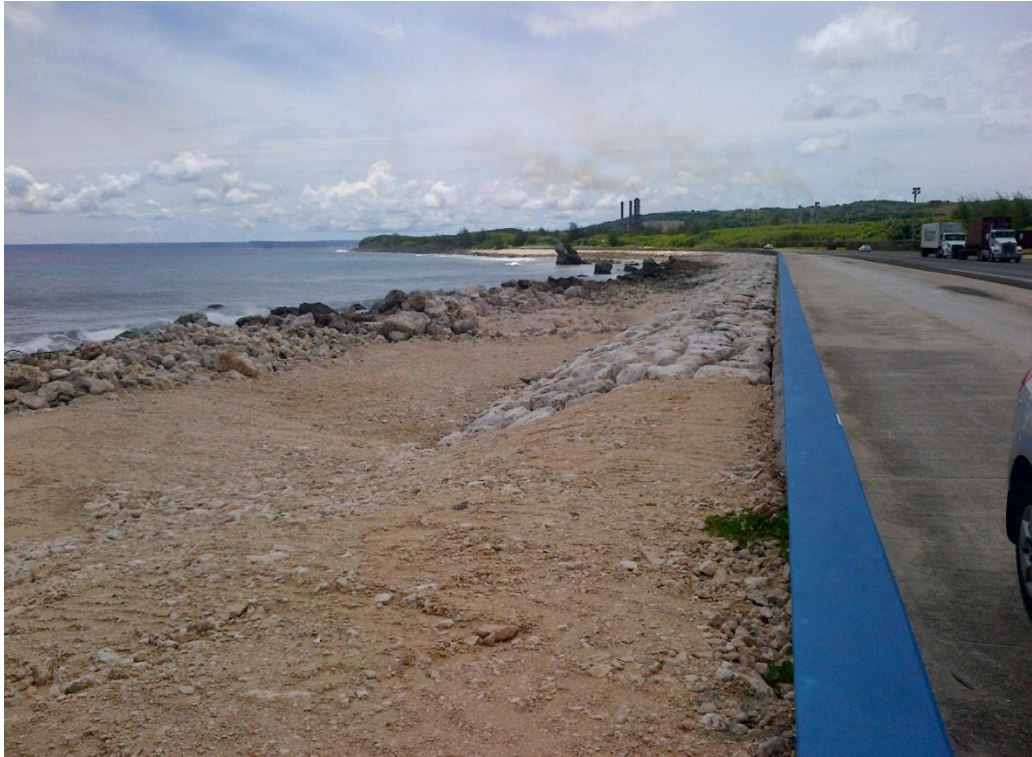
Photo Description: DPW Seawall project looking east from the project ending point. The project was not completed.
