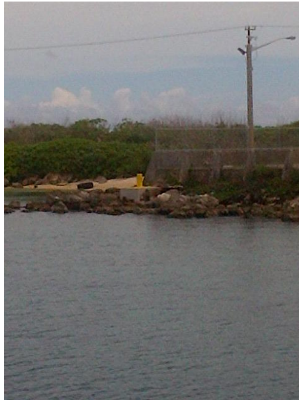
Photo Description: Shore bollard behind Cementon north of the western mooring dolphin looking northwest from the western breasting dolphin.
