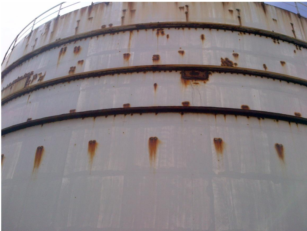
Photo Description: Western wall of Tank 1 looking east.
