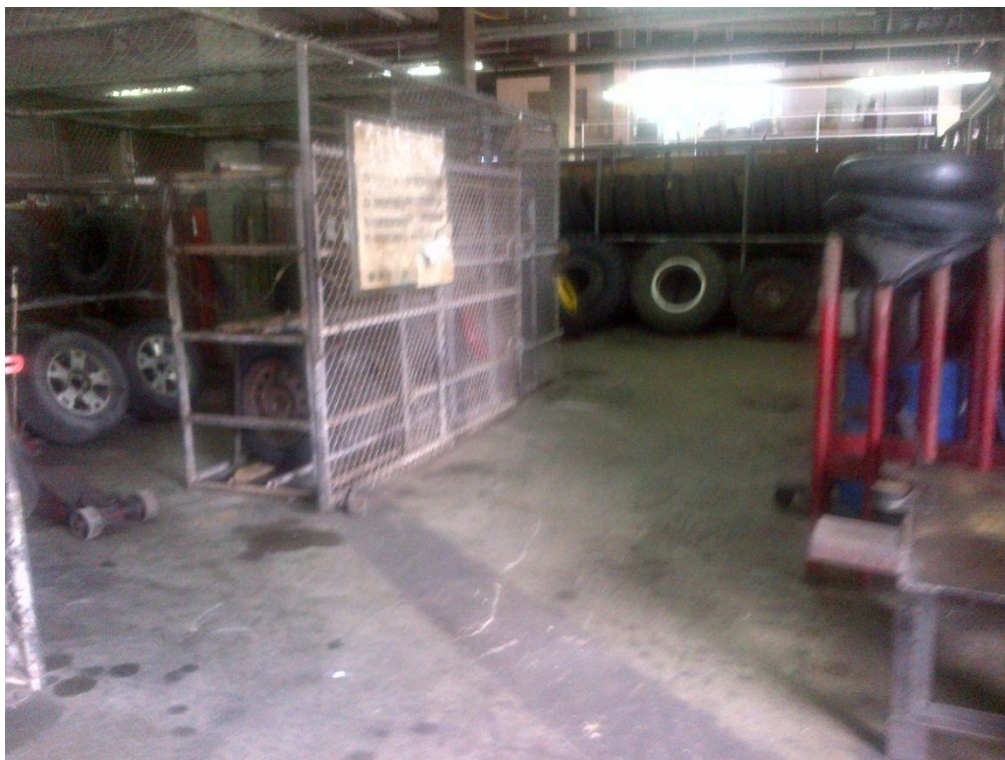
Photo Description: Tire shop area within EQMR facing east.
