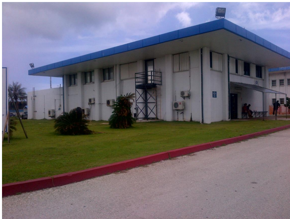
Photo Description: Administration Building Annex looking southwest.
