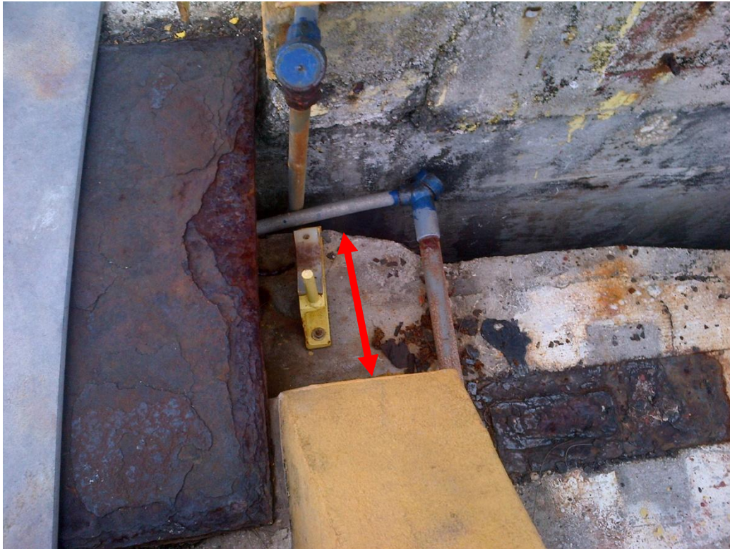
Photo Description: The shift away from the shore as seen on western side at pier.
