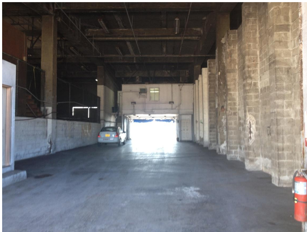
Photo Description: Bay 2 of Warehouse 1 looking south.
