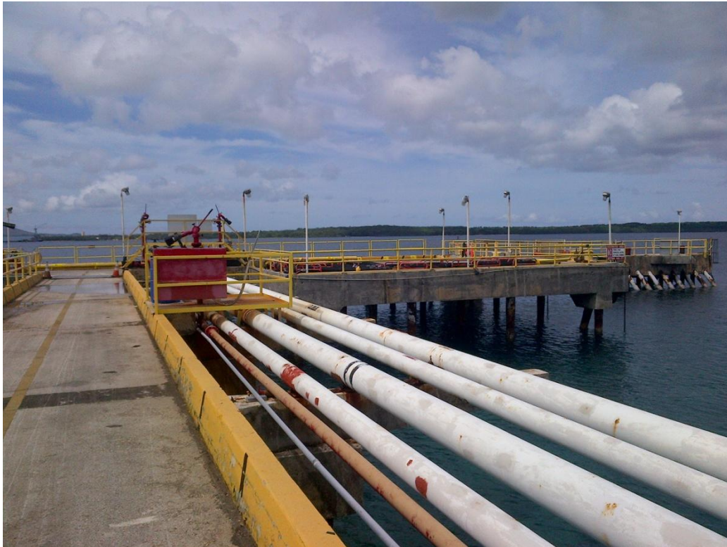
Photo Description: Golf Pier western half looking south.
