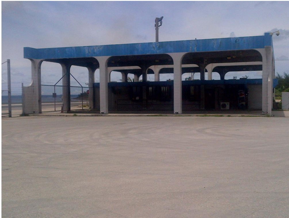
Photo Description: Gate Administration Building and canopy looking east.
