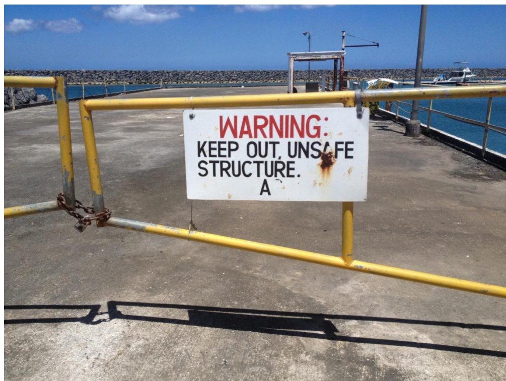
Photo Description: Gate on top of elevated pier blocking vehicular access.
