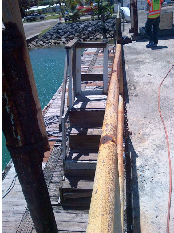
Photo Description: Boat dock/ float located on north side of elevated pier looking east. Stairway is of wood construction and in very poor condition.
