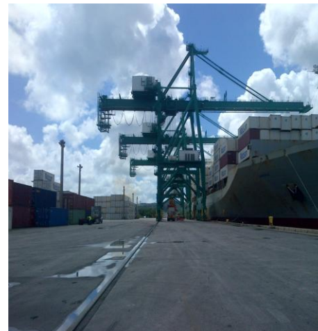
Crane Rails at F-4, F-5 and F-6
