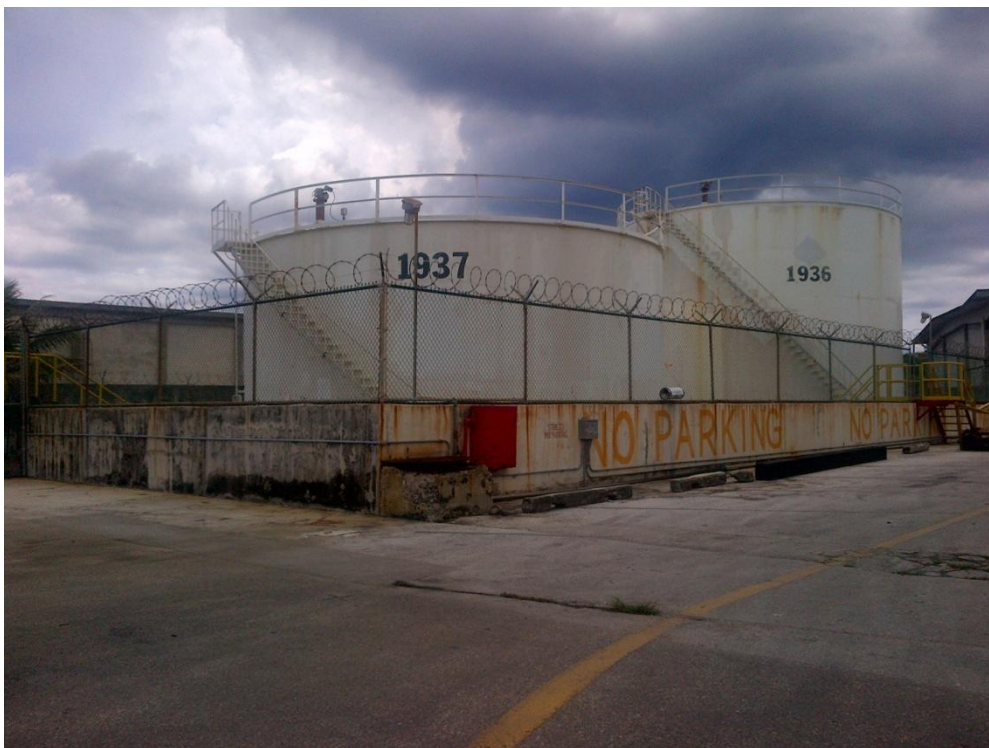
Photo Description: F-3 Fuel bunker west of Warehouse 1 looking north.
