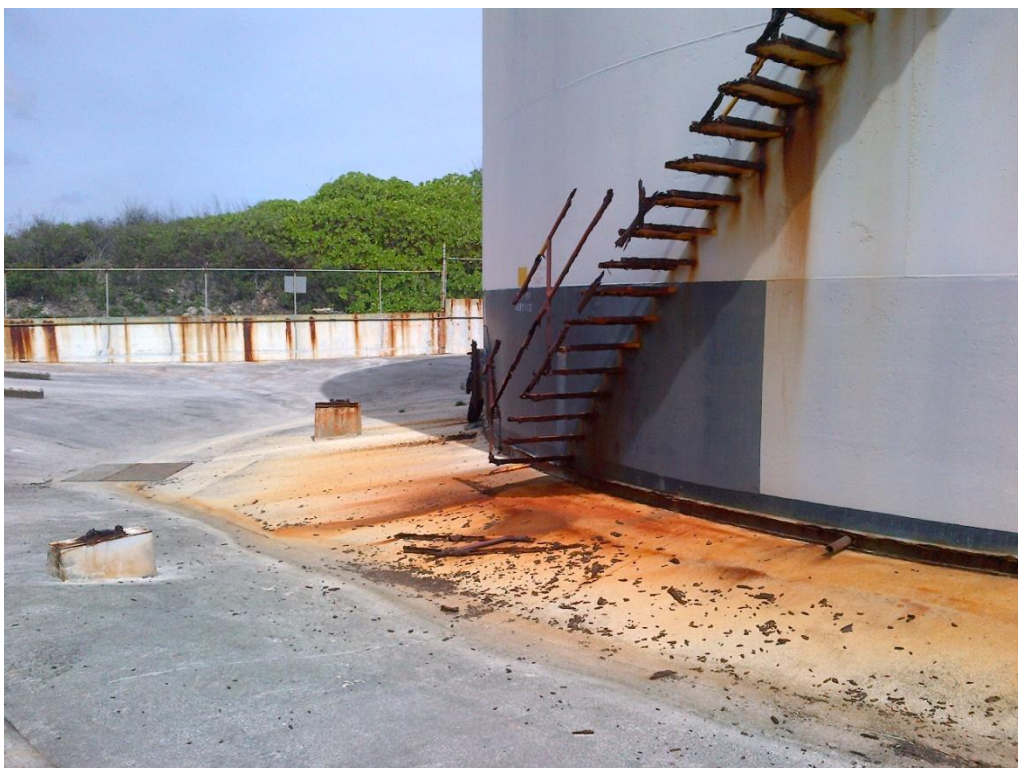
Photo Description: Tank 3 stairway looking west.
