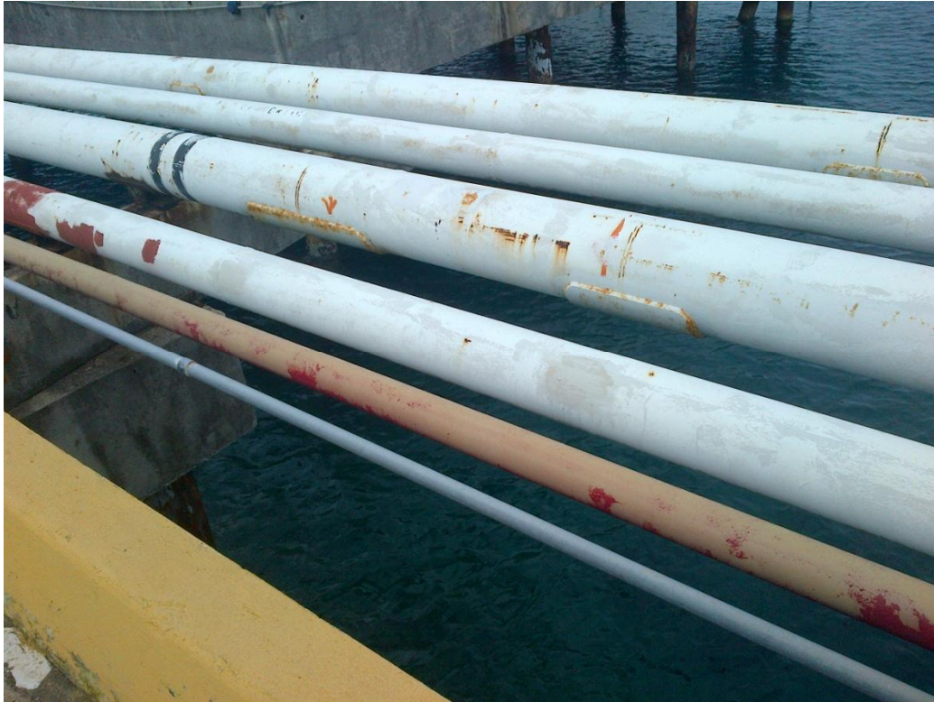
Photo Description: Fuel lines from landside to pier structure.
