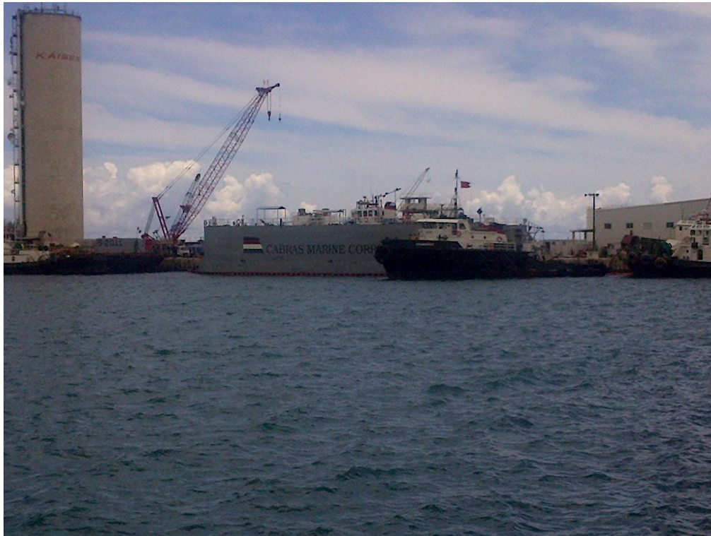
Photo Description: Looking towards F-2 from F-3.
