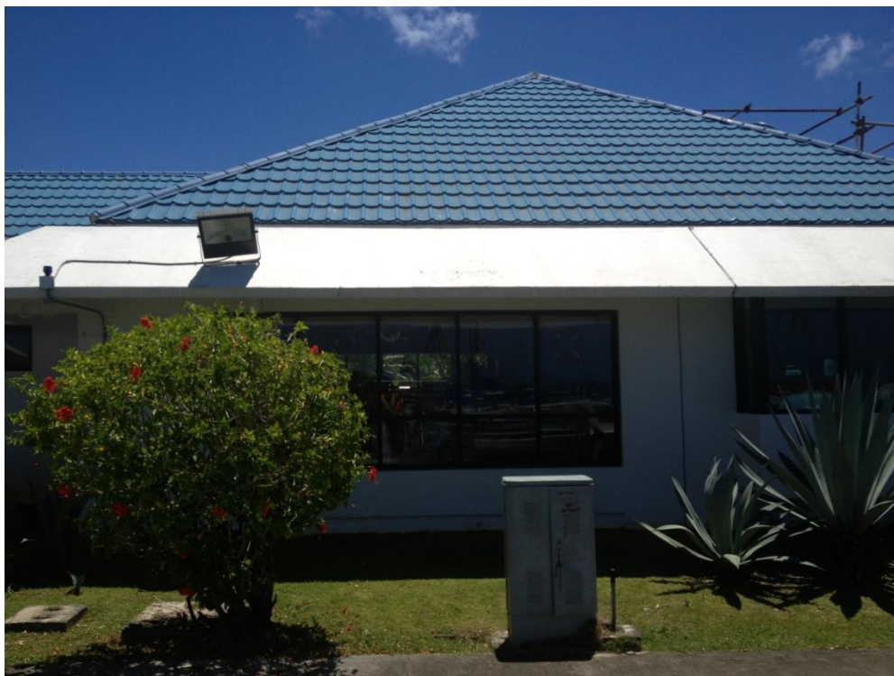
Photo Description: West side of the Restaurant Building looking east.
