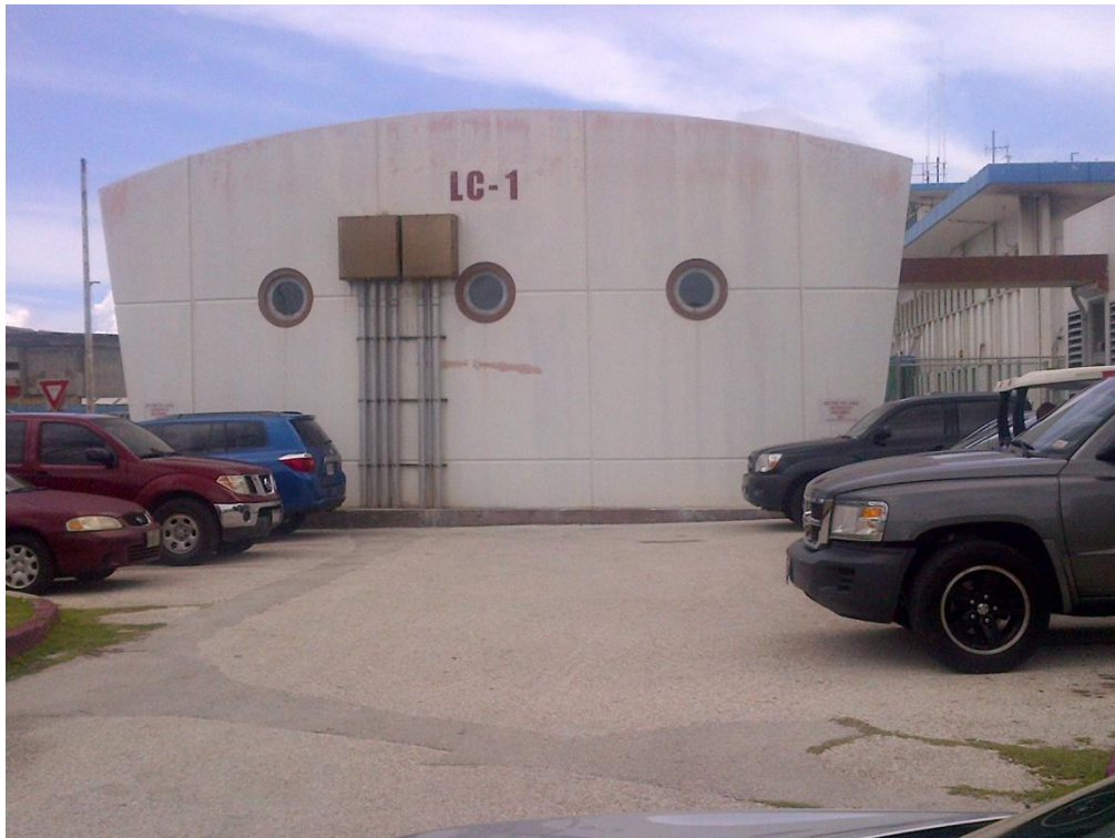
Photo Description: LC1 Switchgear building looking west.
