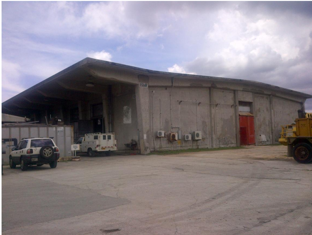
Photo Description: EQMR Building looking north.
