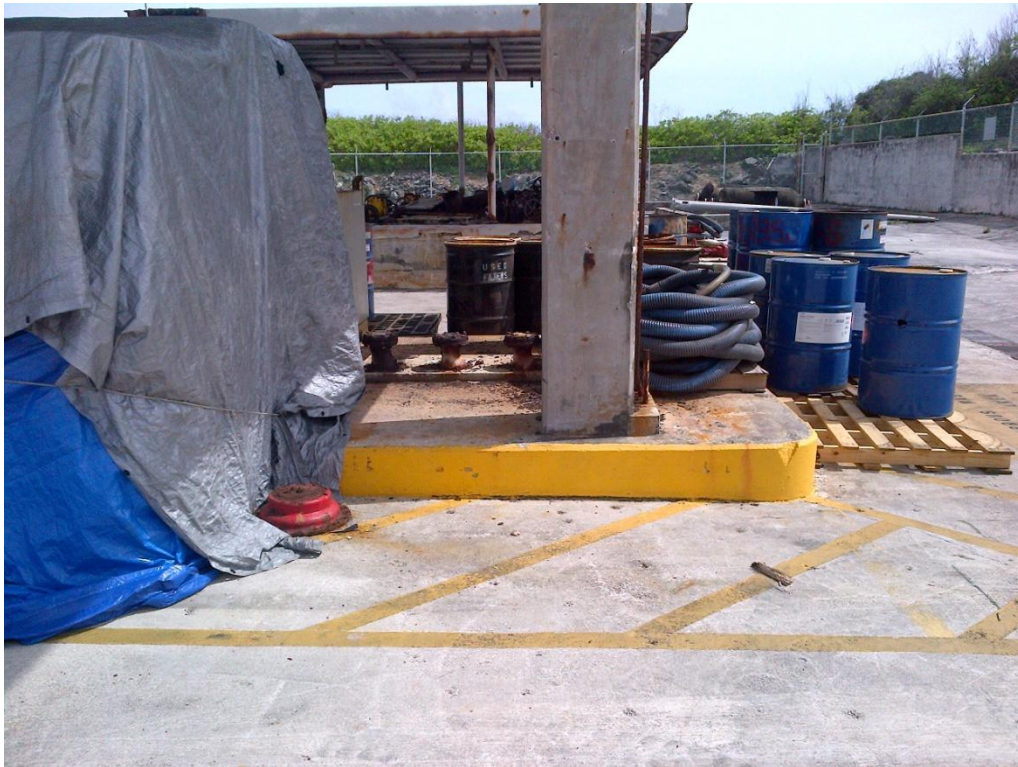
Photo Description: East end of the loading rack structure looking north.
