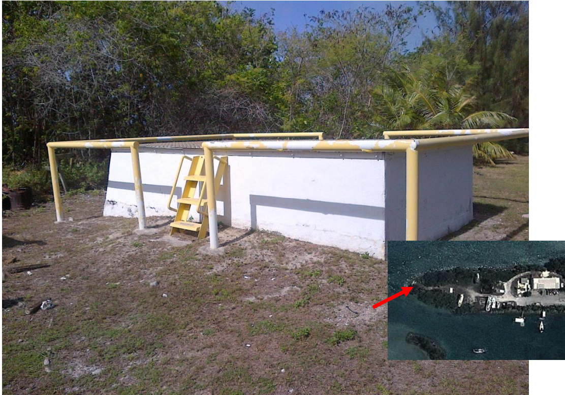
Photo Description: Tristar's Valve pit on the end of the peninsula.
