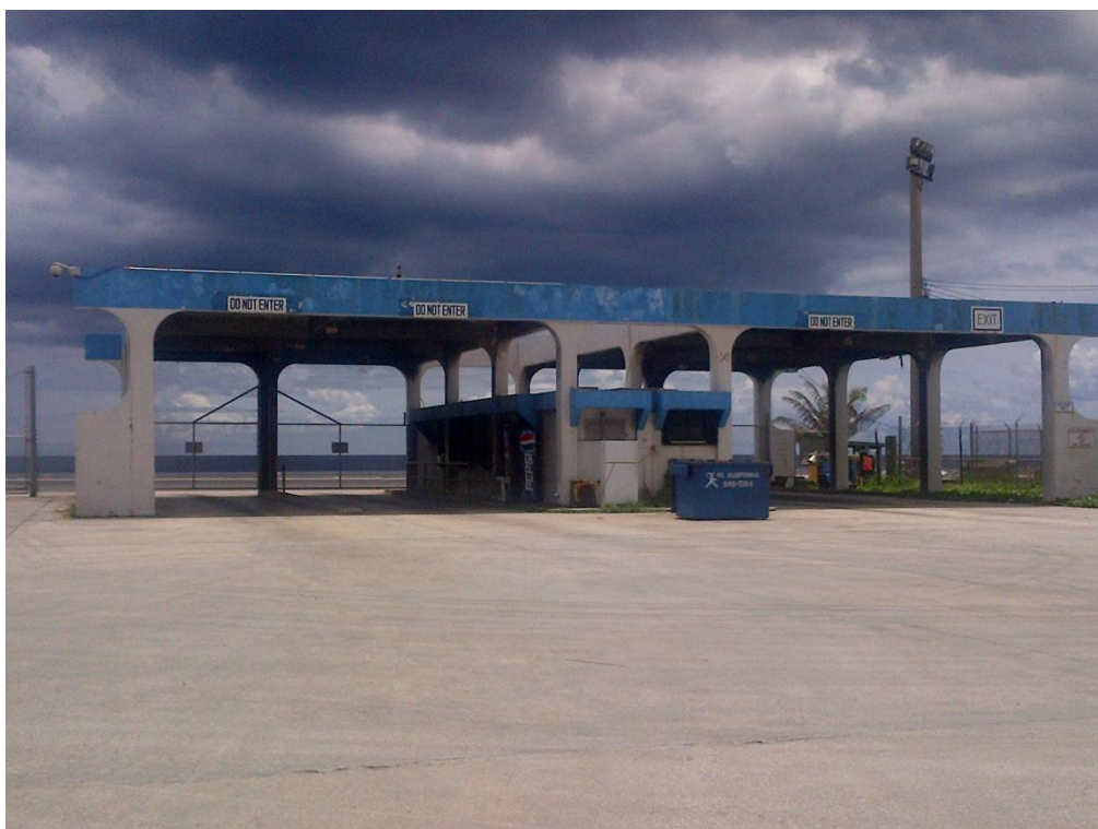
Photo Description: Gate Administration Building looking north.
