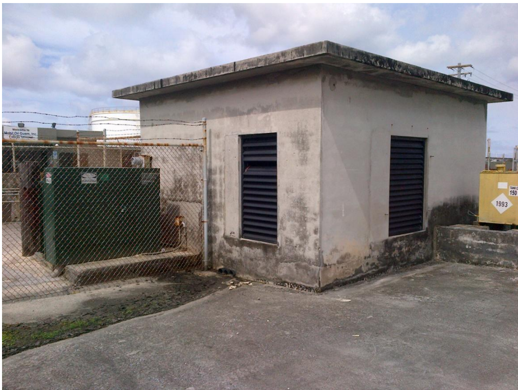
Photo Description: Generator building west of the administration building looking southwest.
