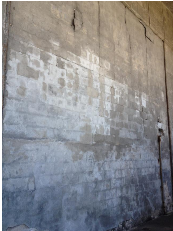
Photo Description: CMU Wall within Warehouse 1.
