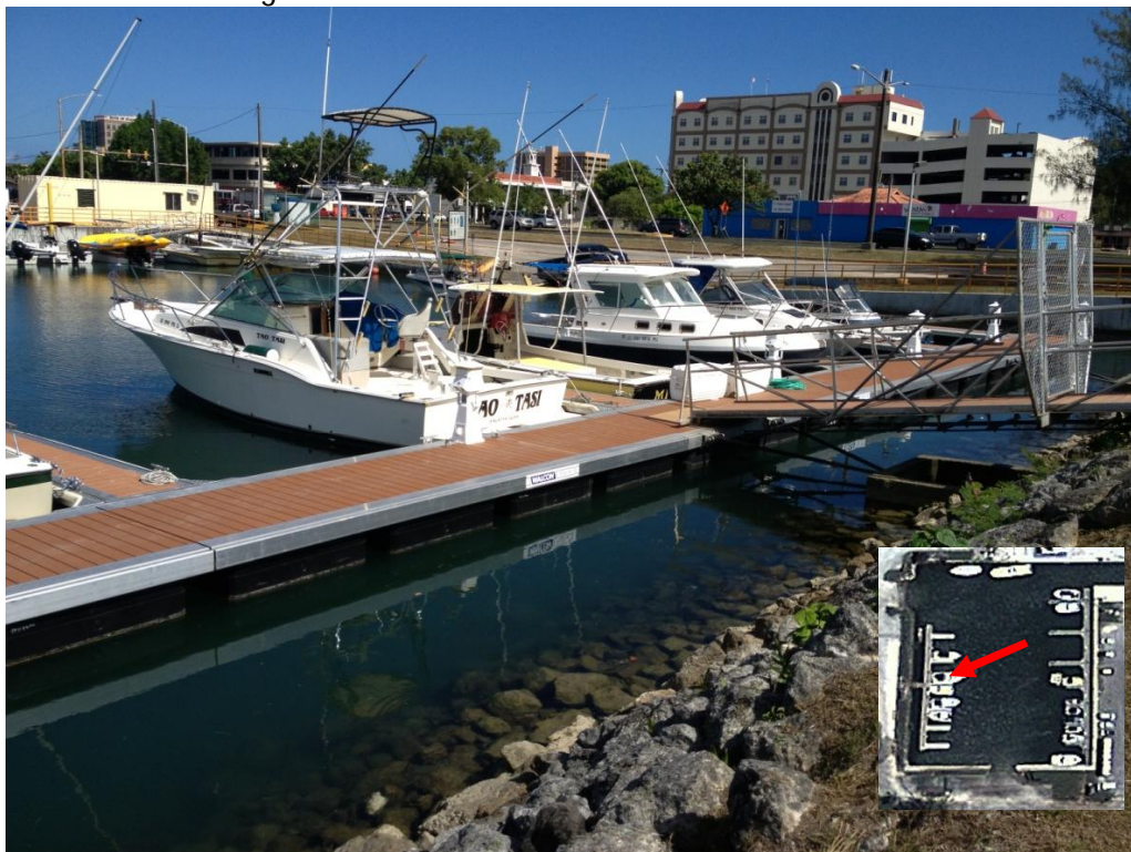
Photo Description: Western boat dock/ float on western edge of west basin of the marina looking southeast.
