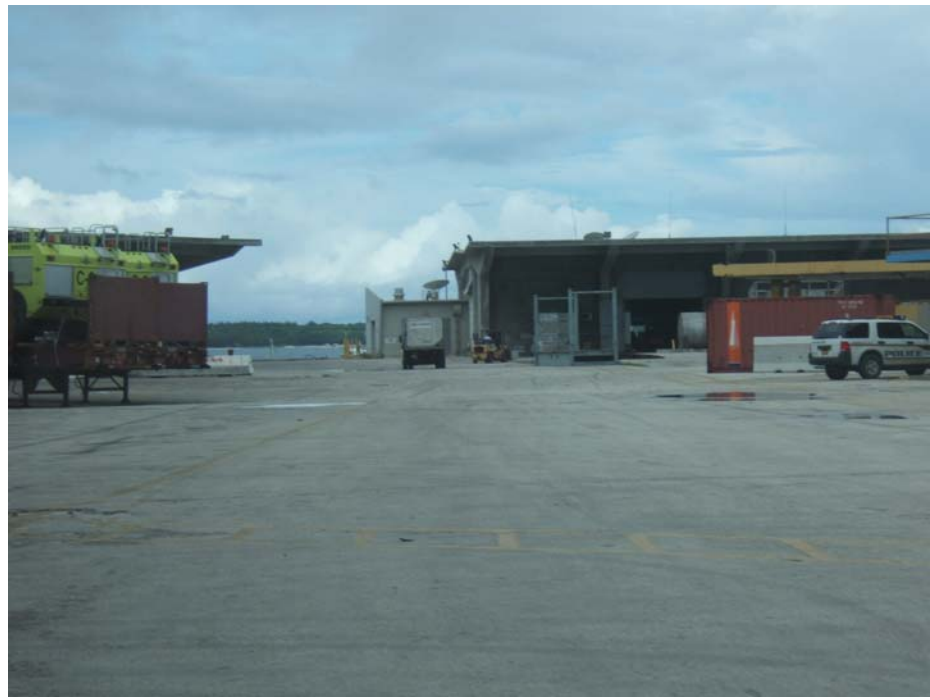
Photo description: W1. concrete paved apron between Shed-1 & Shed-2
