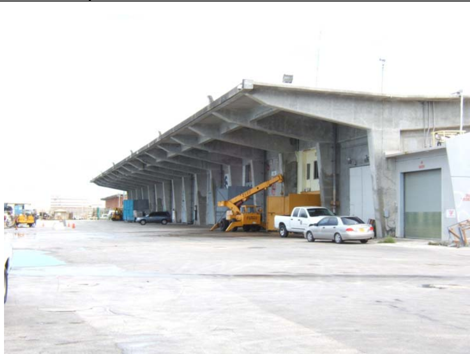
Photo description: W1. side elevation (view from Shed-2 side)
