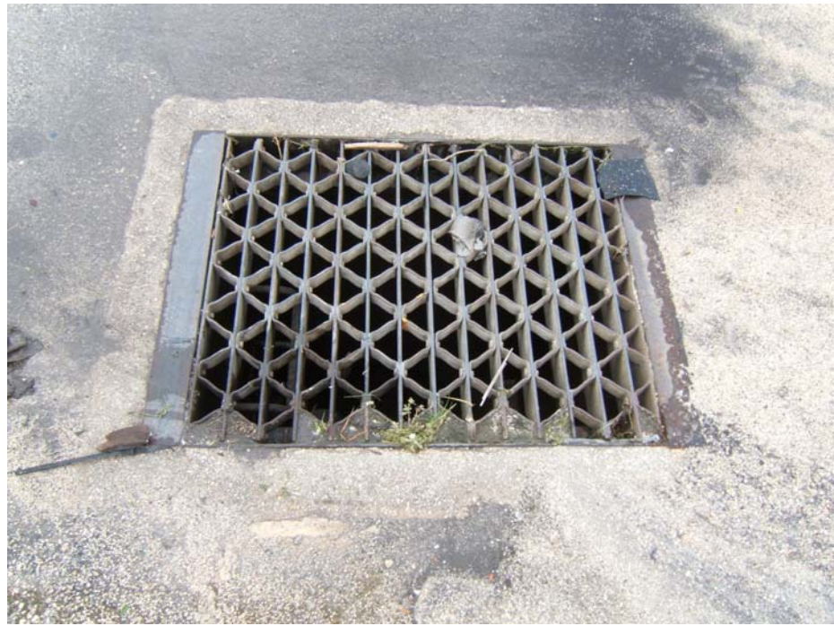
Photo description: Typical drain sump (near abandon gas station)
