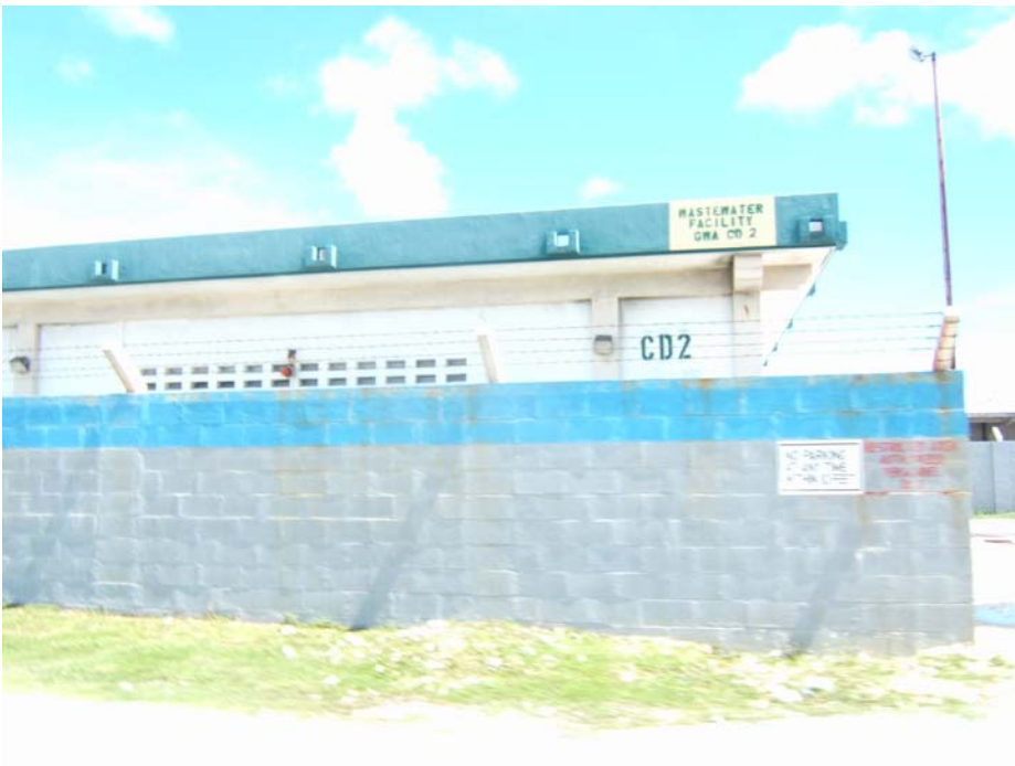
Photo description: Sewerage Pump House
