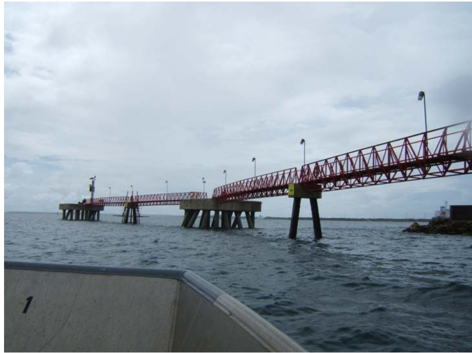
Photo description: connection bridges between decks for F-1, to end of F-1
