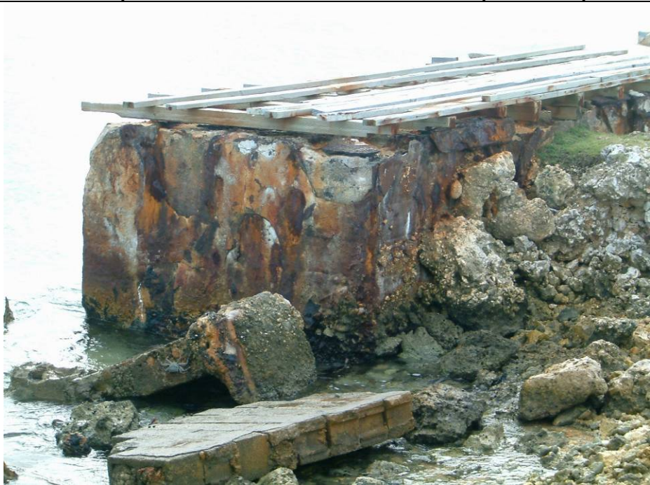
Photo description: View from the land side of Seaplane Ramp
