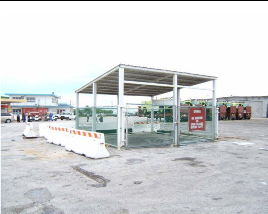
Photo description: Hazard storage (behind W2)
