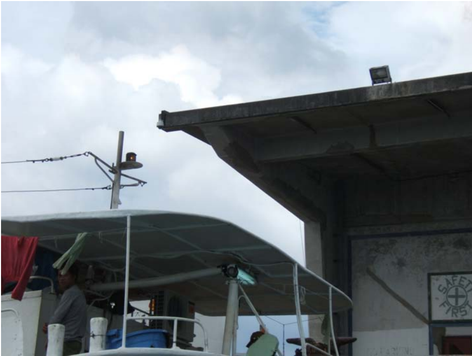
Photo description: W1. cantilevered span canopy
