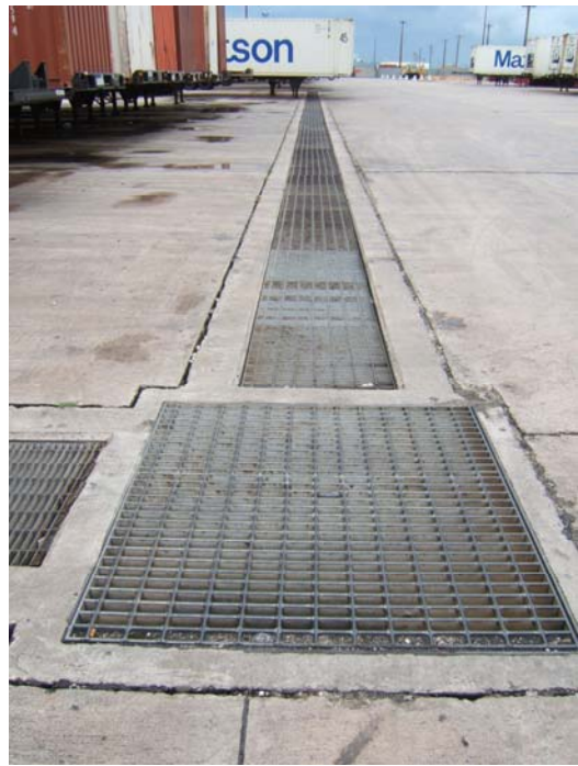
Photo description: Yard Drains – surface ditch & sump pit
