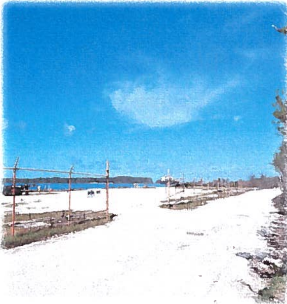
Access Road to "H" Wharf
