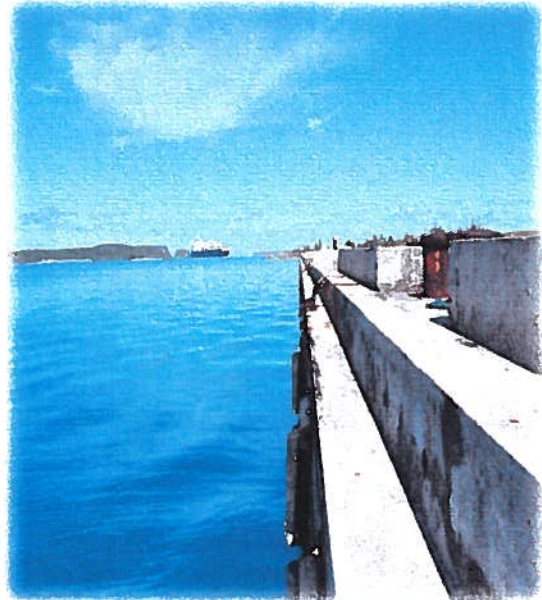
Front of "H" Wharf Structure
