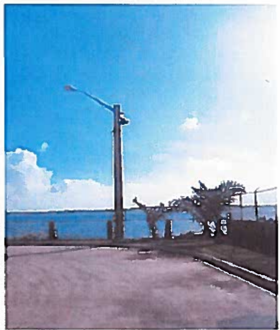
CEMENTON EXISTING LIGHT POLE
