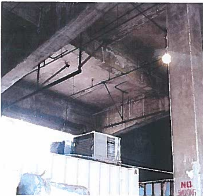
North Side Roll up Door Steel Track to be Remove
