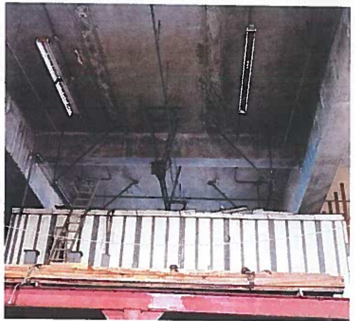
South side Roll- Up Door Steel Track to be Remove
