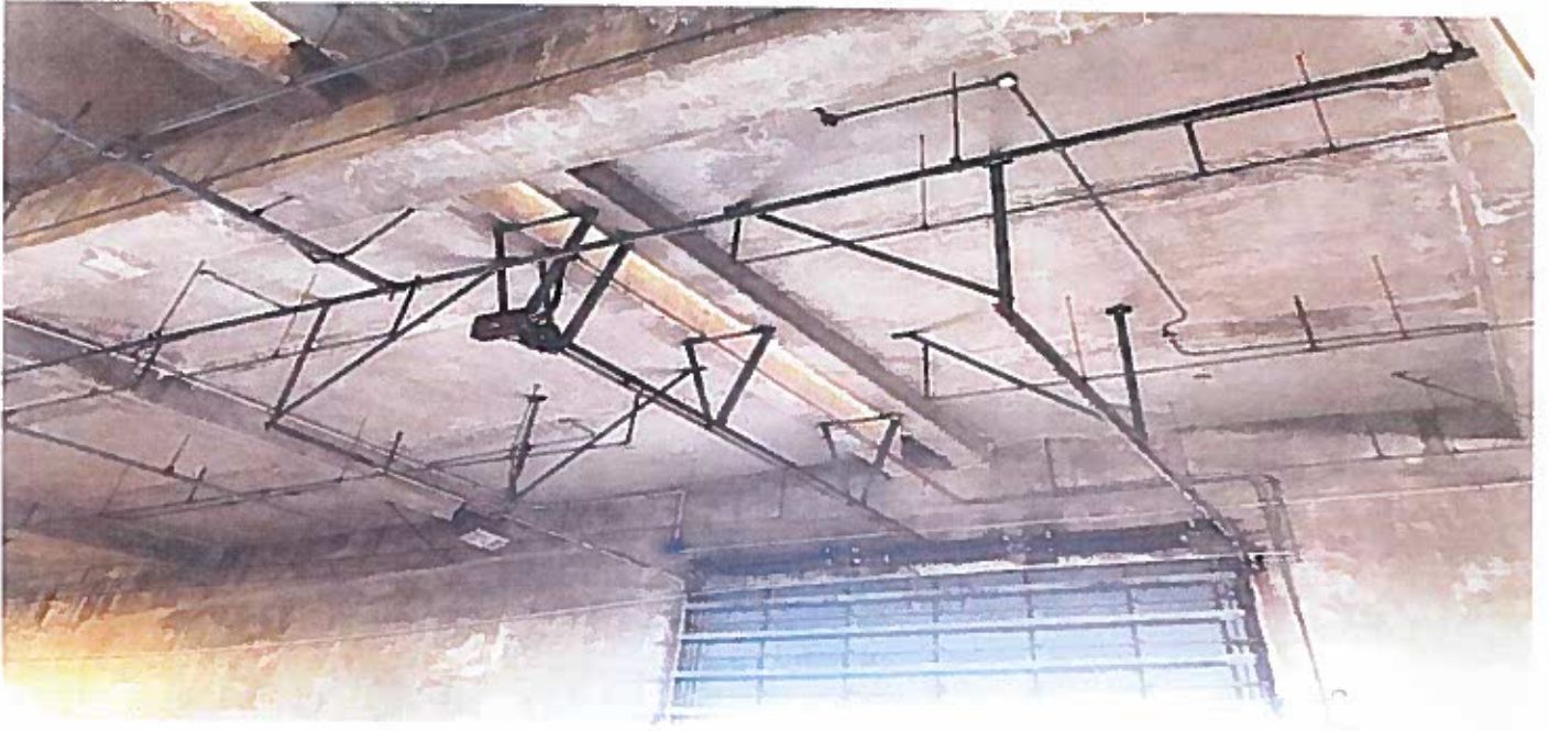
West Side Roll up Door Steel Tracks to be Remove
