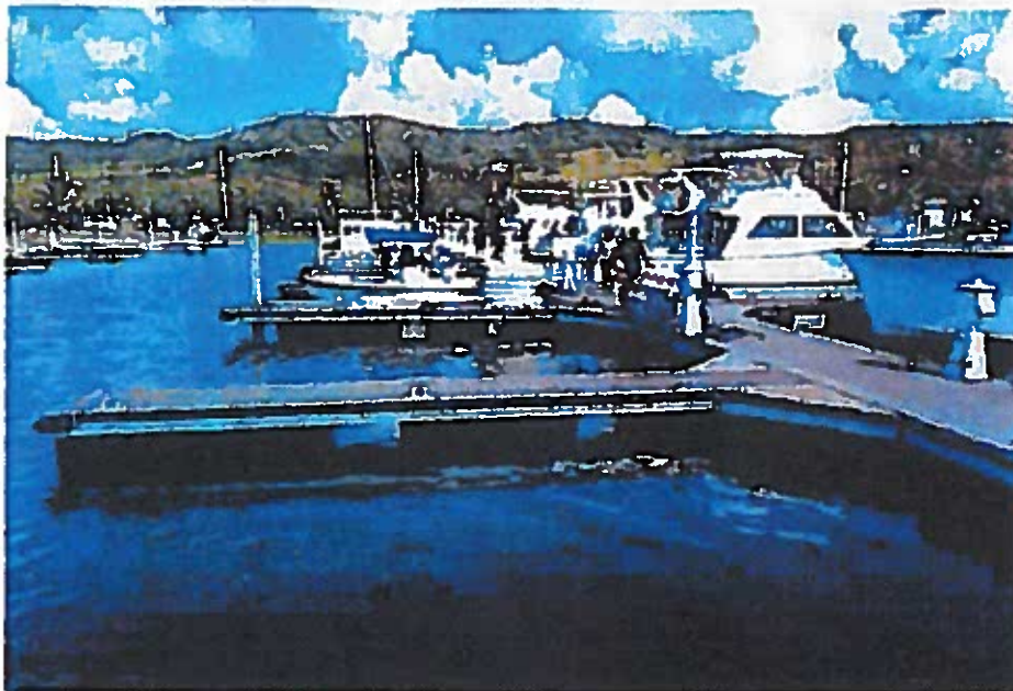
View of typical slip with utilities stub.
