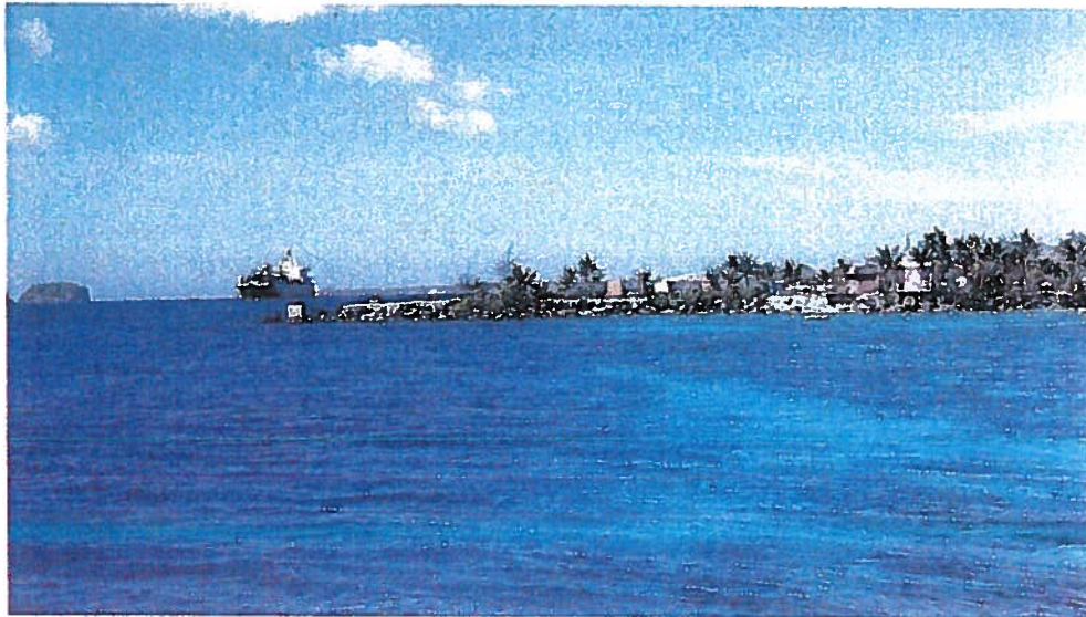
Photo 1. East pier of Dog Leg Pier, facing west, March 2019.
